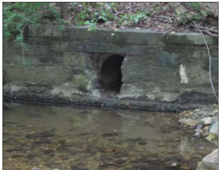
Runoff from roads, parking lots, and other hard surfaces "disappears" into the sewer system through gutters and drains that lead directly to creek outfalls, such as this one.
