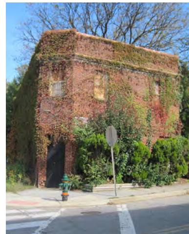
Chesapeake House could be renovated for partner use or historic leasing.
