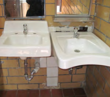
Park restrooms should be updated as needed, including use of water-saving fixtures to prevent running faucets such as this one.
