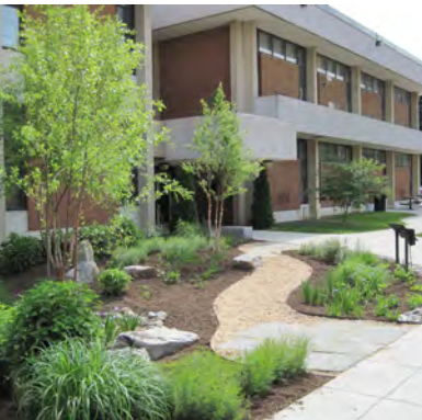
Rain gardens such as this one capture rain near where it falls. (before installation, top, after installation, bottom)
