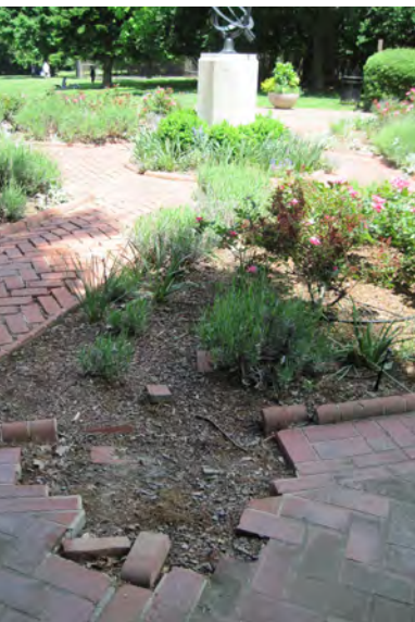
Montrose Park has ongoing maintenance needs.
