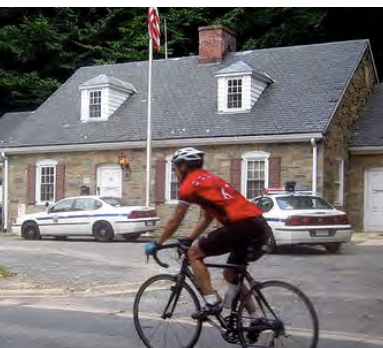
The Lodge Building currently houses a substation for the U.S. Park Police.
